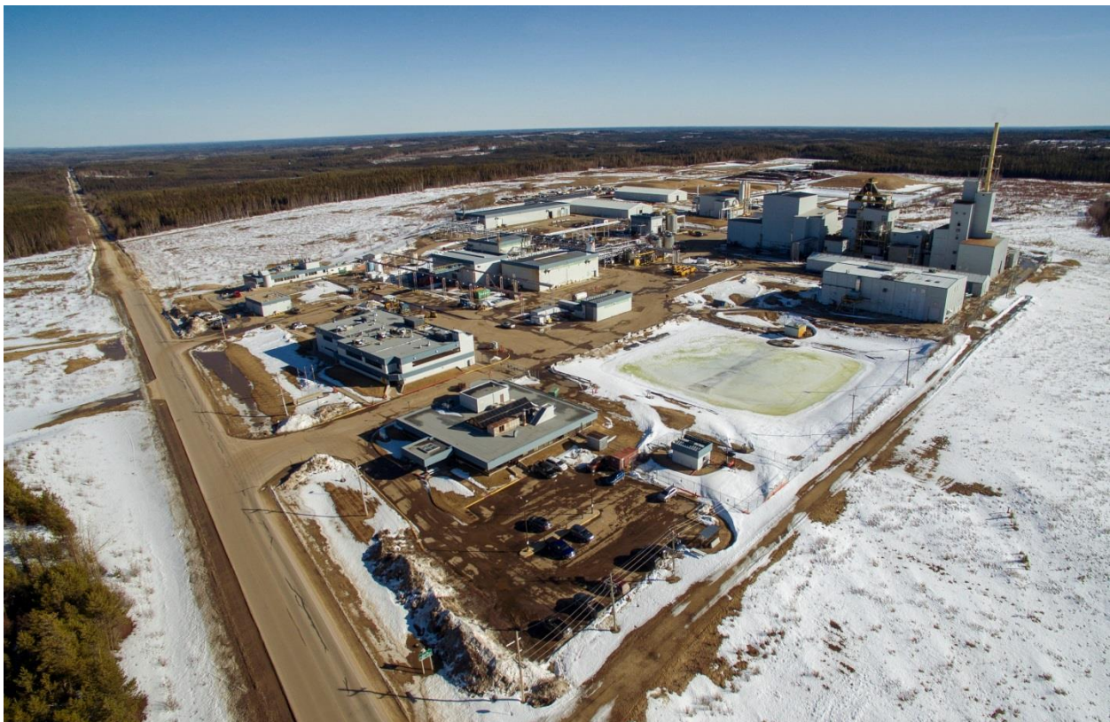
Figure 1-1: Swan Hills Treatment Centre
