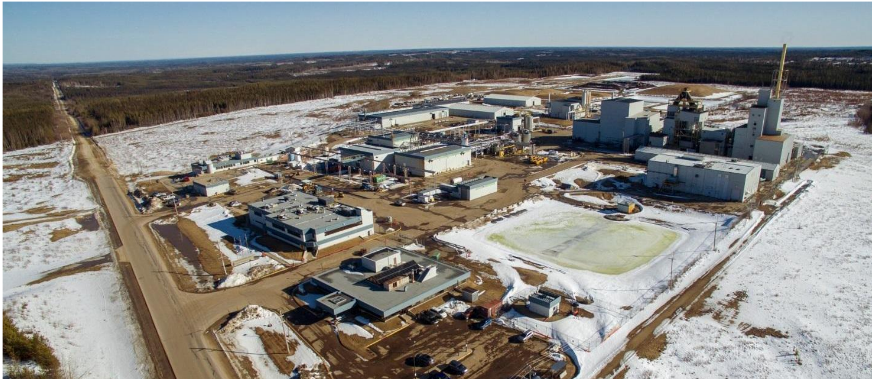
Figure 1. Swan Hills Treatment Centre Facility
