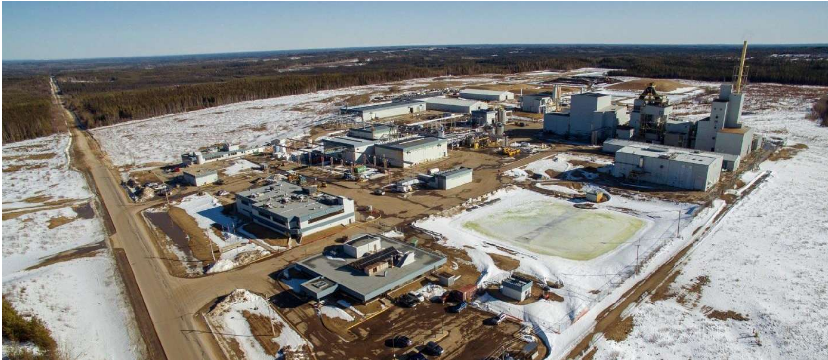
Figure 1. Swan Hills Treatment Centre Facility
